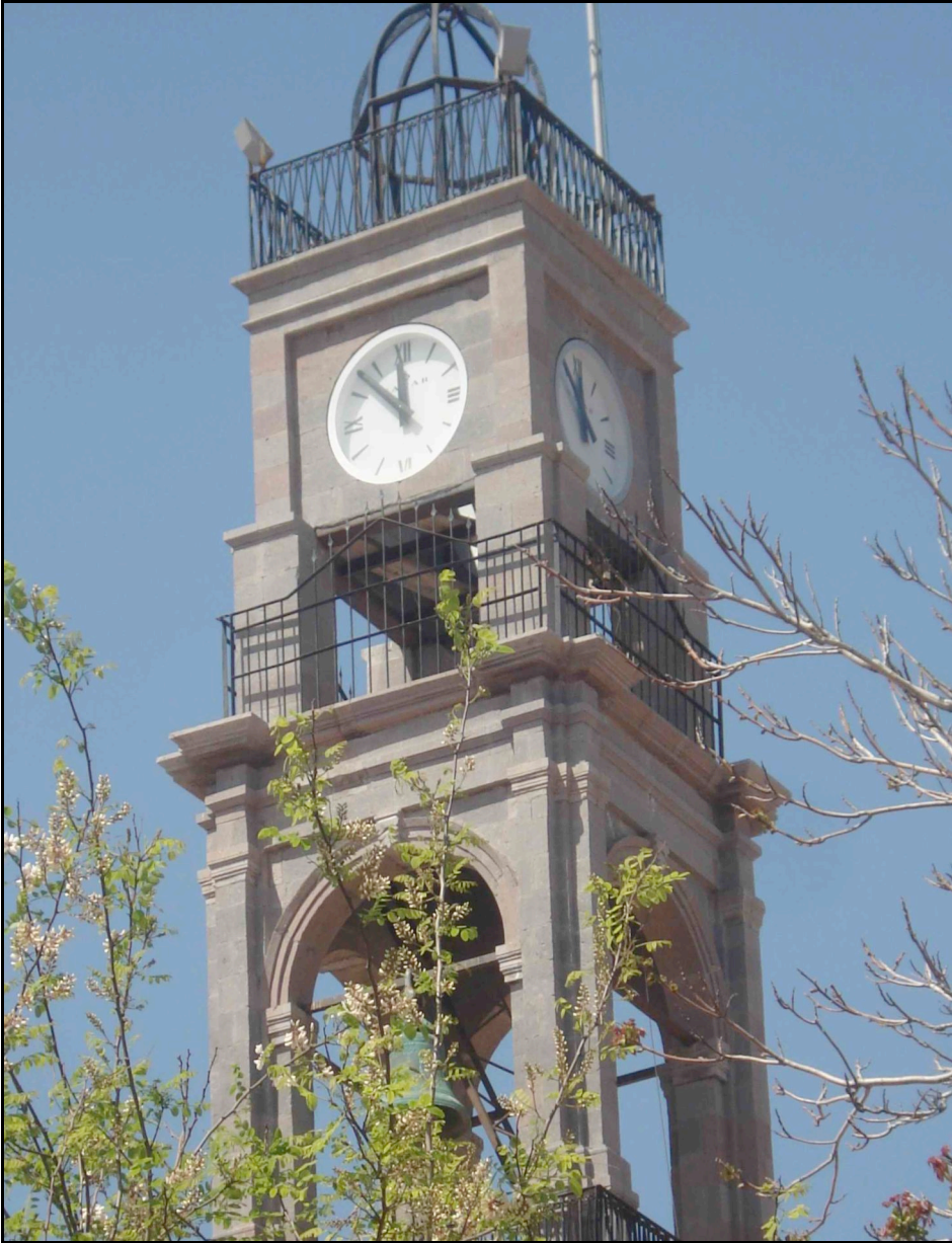
Figure 8 – Four storey clock tower of Panagia Kimisis church, the restoration of which was completed in 2007 with Turkish government contributions (Bozcaada, 2008) (author’s photograph)
